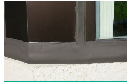
Sealant Joints After
