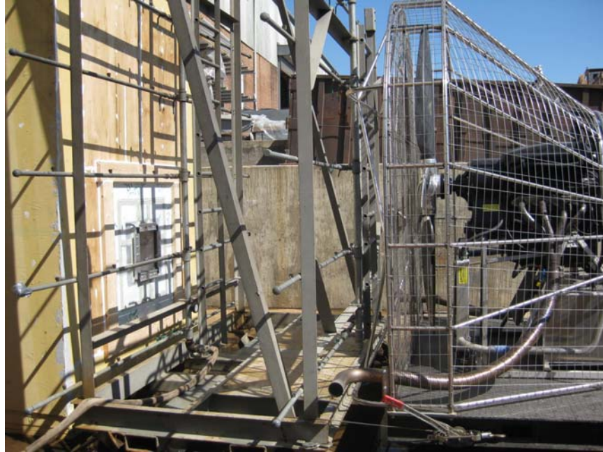
Photo No. 3 Dynamic Water Penetration Set-up
