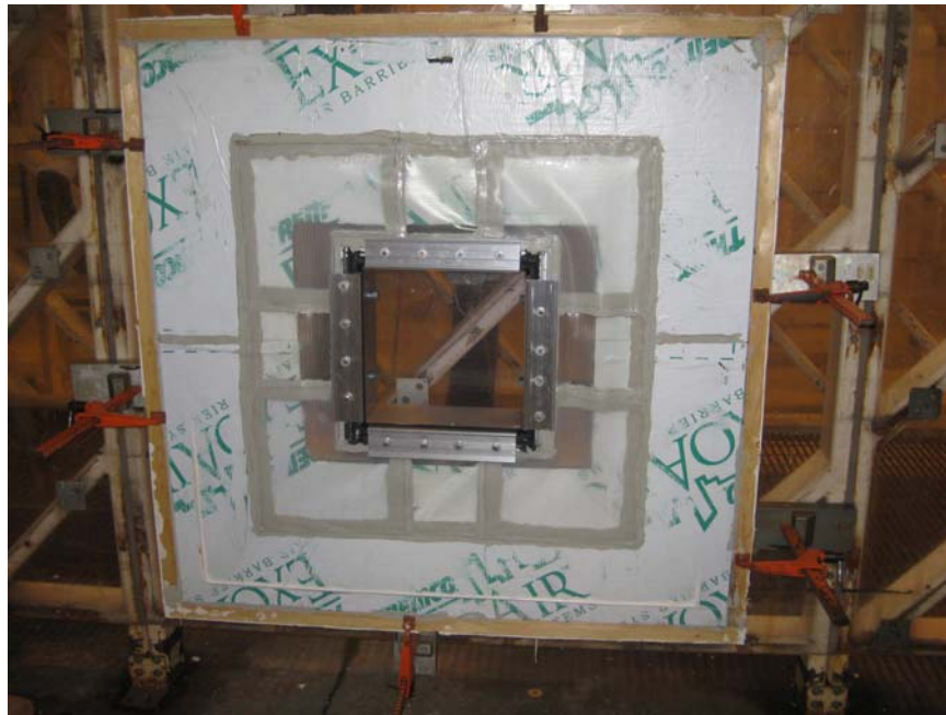
Photo No. 4 Structural Load Set-up
