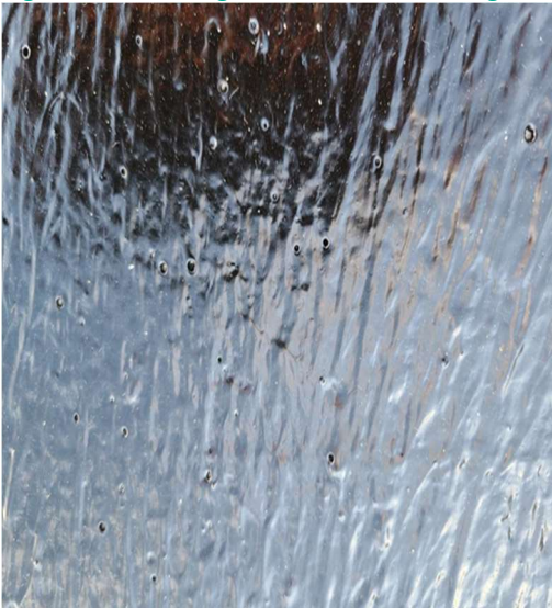
Figure 3 - Pinholing in a membrane during cure
