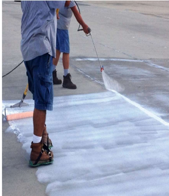
Figure 6 – Priming prior to membrane application to reduce or eliminate pinholing
