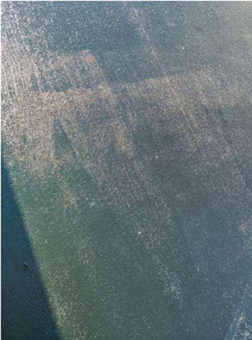
Figure 5 - Creating a membrane “scratch coat” with membrane
