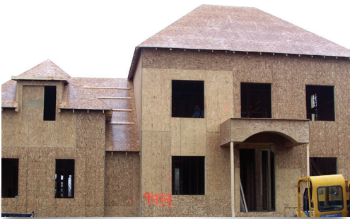
Before Enviro-Dri Weather-Resistant Barrier System
