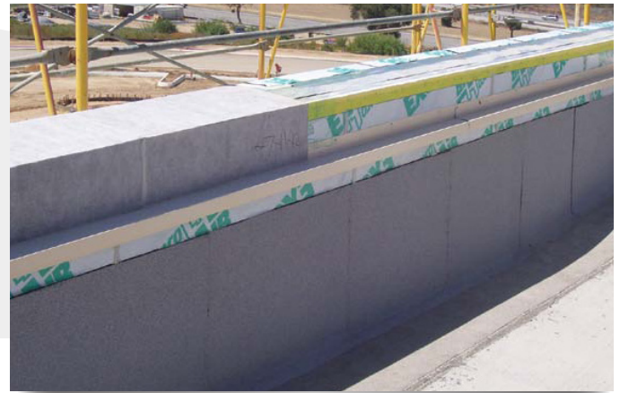
▲ The ExoAir 110 Self-Adhered Air & Vapor Barrier Membrane is carried over the parapet and the ExoAir HTF is applied over it to connect them, providing continuity from the roof to wall.
