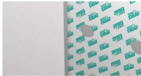
Ref 2 – Insulation installed
