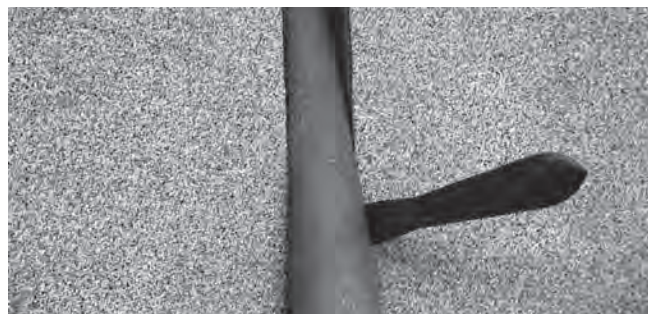
FIGURE 7.2 – INSERTING BACKER ROD
