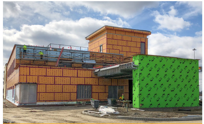
The system results in superior control of air, water and vapor throughout the building envelope.
