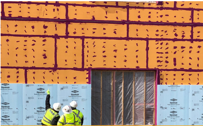
Panels with the air barrier already applied cuts out a step on the installation process.
